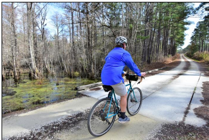
Crossing bridge over swamp on Bossis Rd.
