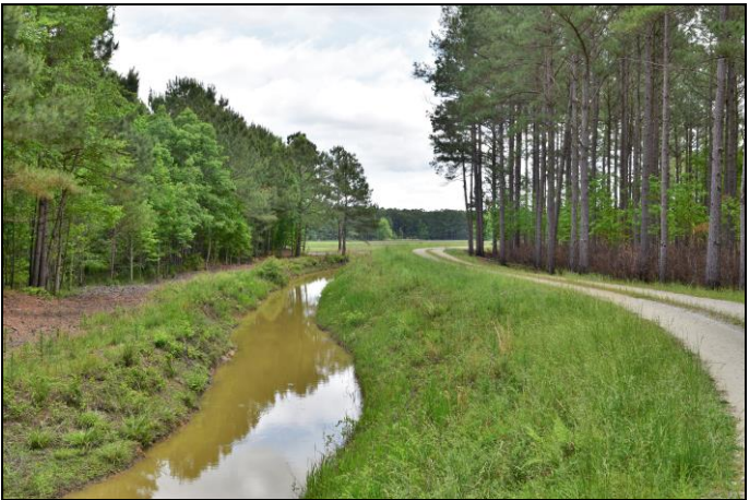
Parts of the trail consist of wide, service roads.
