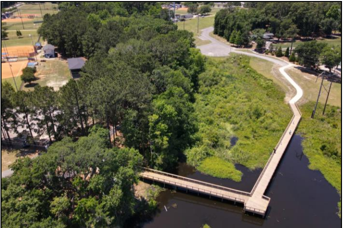
Aerial view of the new boardwalk and dock.
