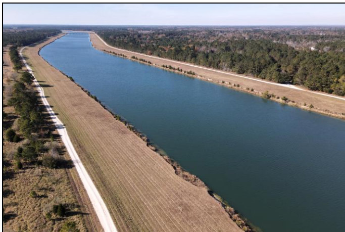
Aerial view of the Rediversion Canal that you'll ride.
